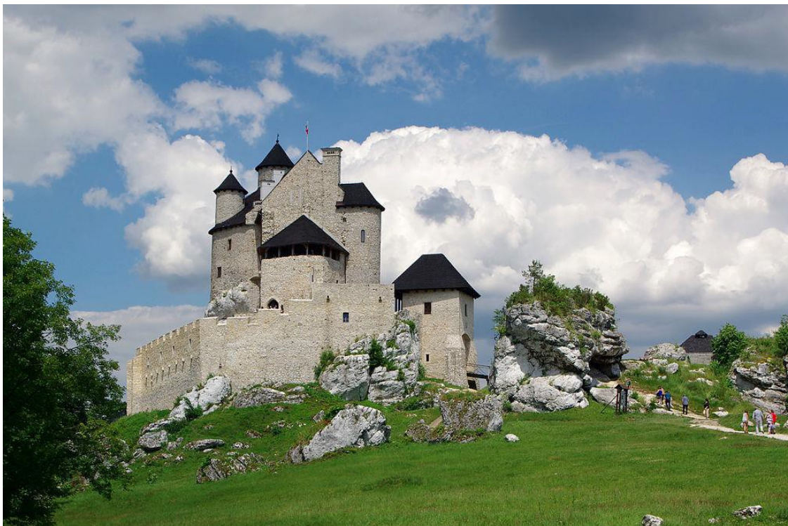
Castle in Bobolice after refurbishment (“reconstruction”).
