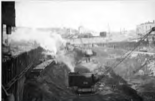
Construction of the bunker
