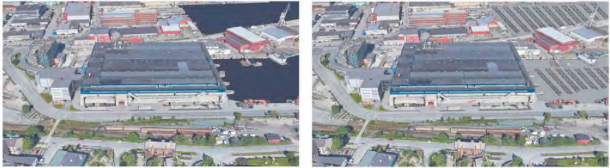
Figure 7. Dora bunker far away from the sea (Google Earth 3D view).
